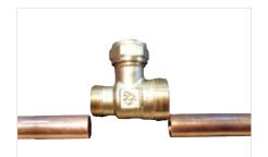
Cut a length of pipe equal to the body of the T-piece. Bear in mind that the body of the T-piece will slide over the pipe to a depth of some 13mm. The T-junction will therefore be positioned 13 mm closer to the cut pipe end.
